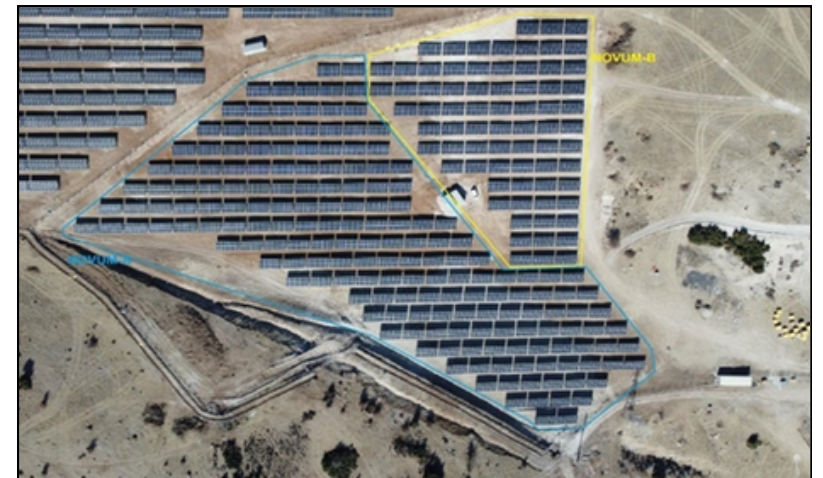
Novum Garden Side Hotel Solar Power Plant
